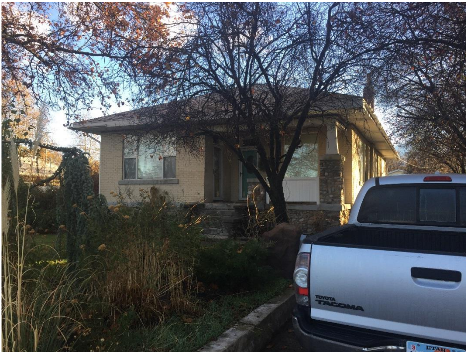
View of Northern parcel (3075 South 900 East), with home to be demolished for Phase 2.
