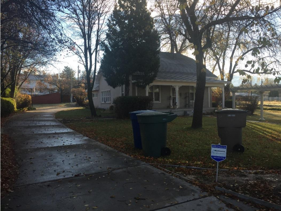
View of Northern parcel (3089 South 900 East), with home to be demolished for Phase 2.
